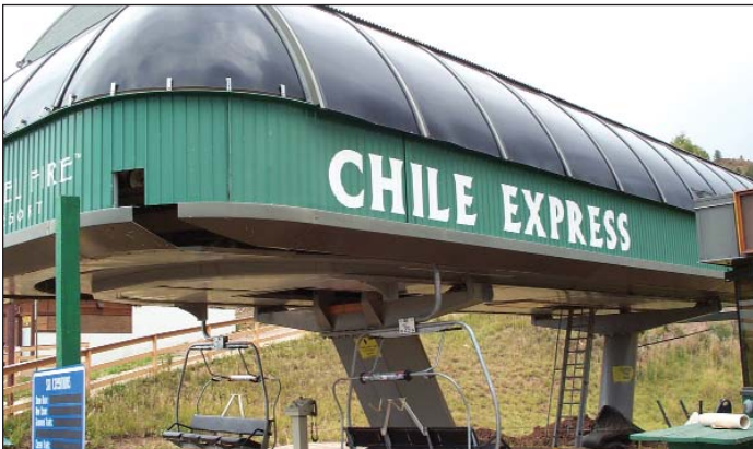
Figure 1. Angel Fire Ski Resort's 10,000-ft (3,000-m) Chile Express chairlift is one of the longest in North America. The lift's path up the mountain can be seen on the cover; its lower terminal station is shown here. The high-speed quad lift can carry 1,800 passengers per hour at speeds as high as 1,200 ft/min (366 m/min). When power quality problems damaged the computers and sensors that control the lift, it repeatedly shut down. Annoyed customers packed up and went home.
